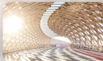
Atyrau Bridge Astana
